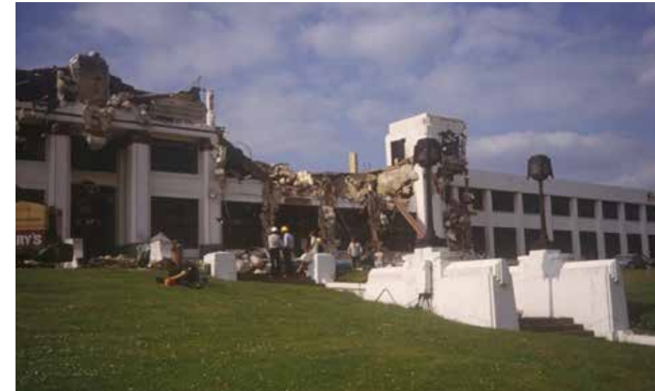
Fig 2.10 Demolition of the Firestone factory in 1980
