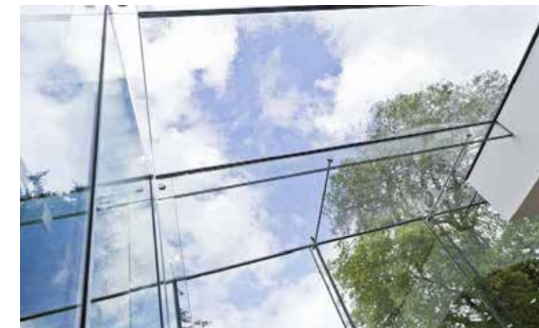
Fig 4.13 Structural glass box
