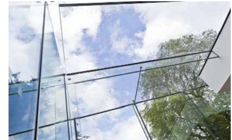
Fig 4.13 Structural glass box
