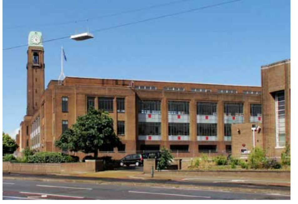
Fig 2.4 Former Gillette factory, built 1937
