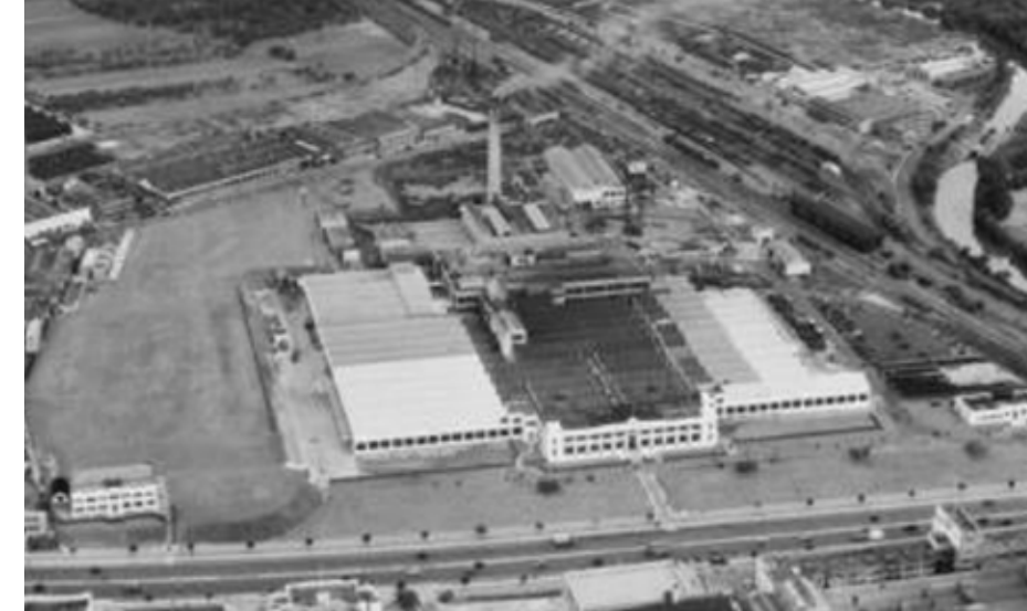
Fig 2.9 Aerial view of the Firestone factory c.1953
