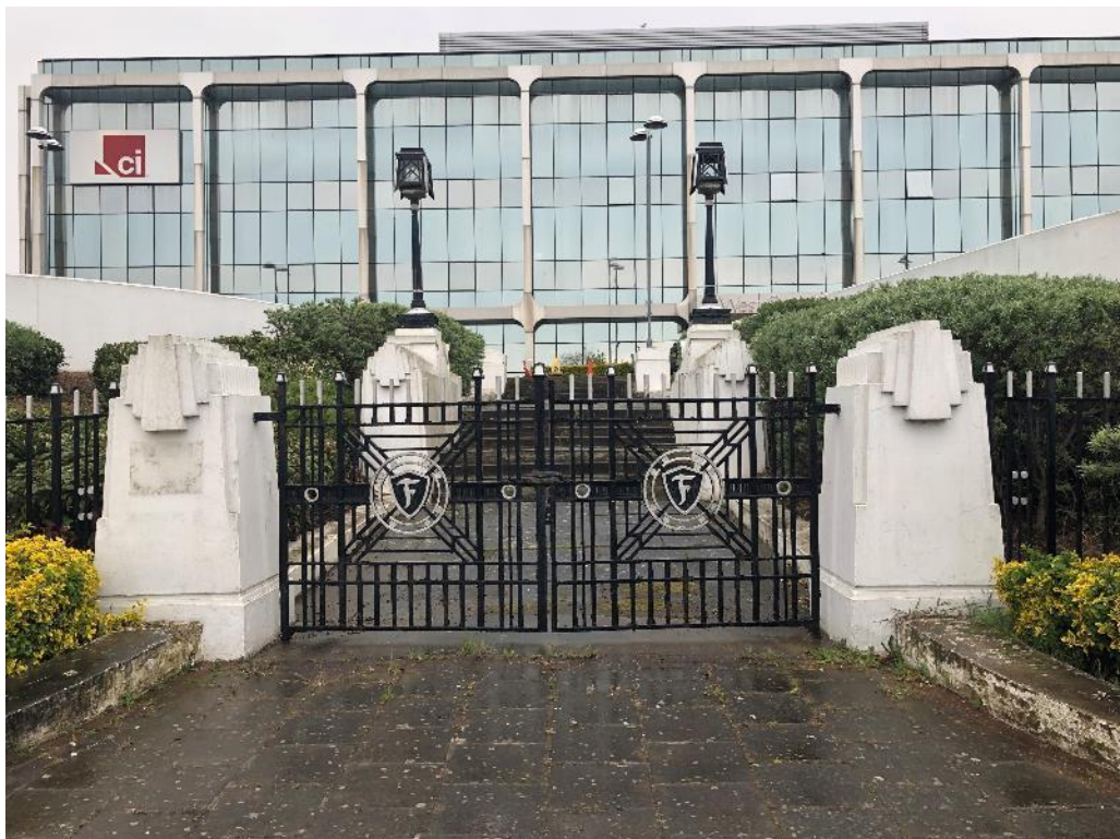
Figure 4.2: Detail of gates and piers to the former Firestone Factory
