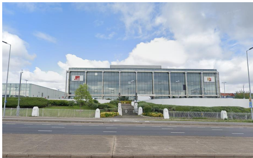
Figure 5.4: West Cross House, viewed from the Great West Road
