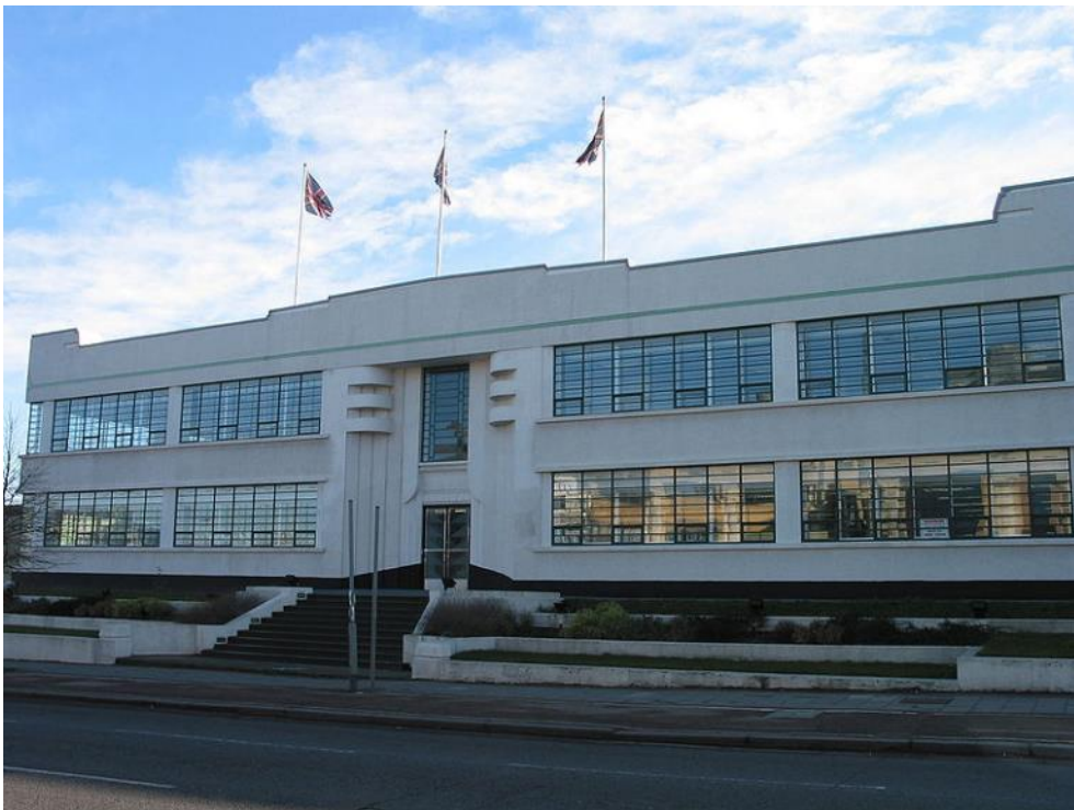
Figure 4.7: Former Coty Factory Premises
