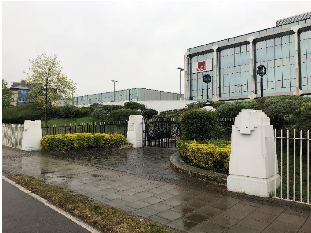
Figure 4.1: Gates, Piers and Railings to the former Firestone Factory, viewed from Great West Road
