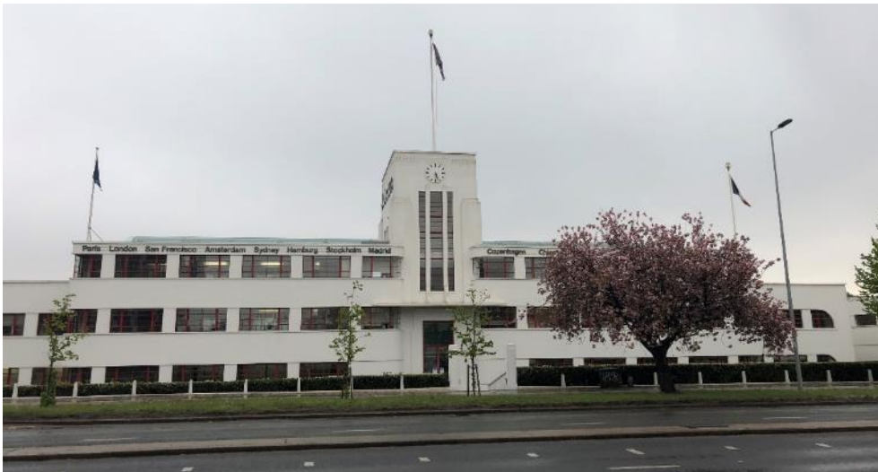
Figure 4.6: South face of 991, Great West Road
