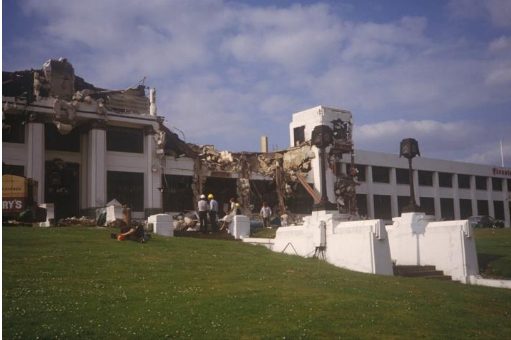
Figure 3.10: Demolition of the Firestone tyre factory in 1980.
