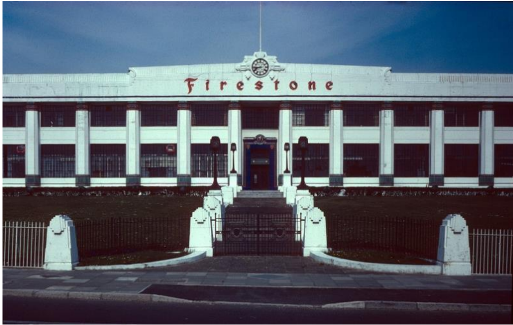
Figure 3.9: Firestone Building prior to demolition.
