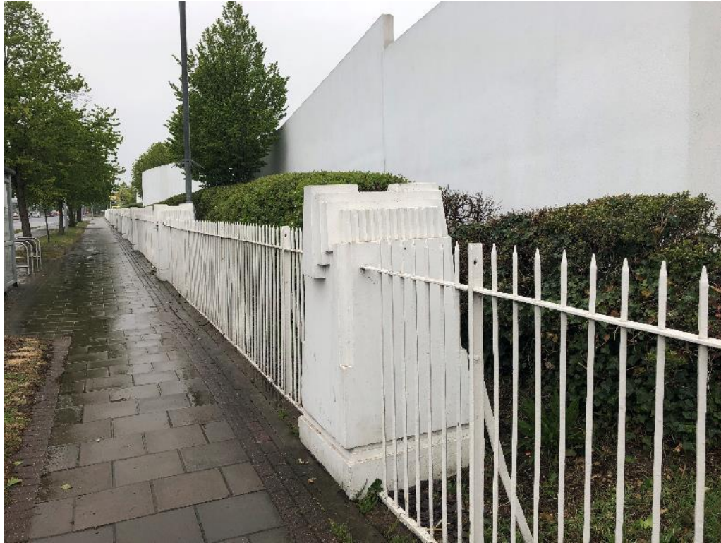
Figure 4.4: Additional railings and piers fronting the Great West Road
