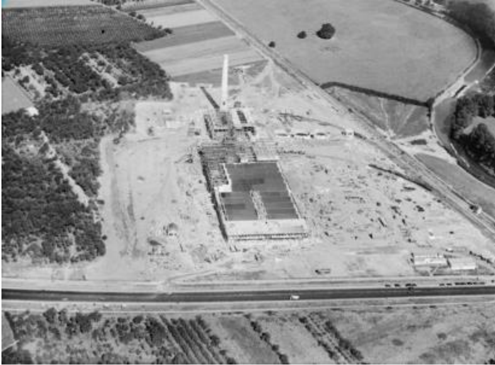
Figure 3.4: Aerial photo of the Firestone Factory under construction c.1928 ( https://britainfromabove.org.uk/en/image/EPW023233 )
