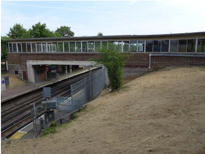
View looking North of existing Overbridge viewed from Public footpath.
