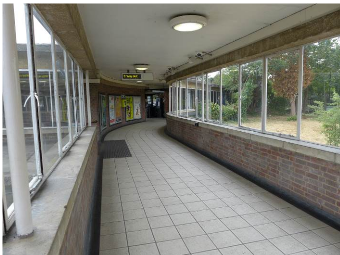
View looking South East along existing Overbridge.
