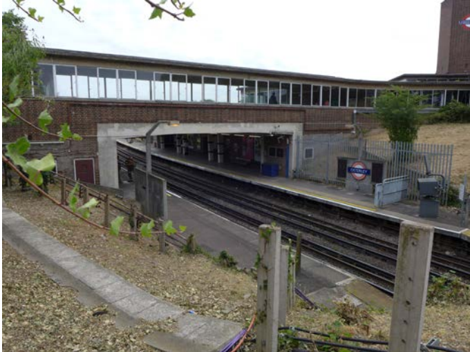
View looking East indicating both platforms and embankment.
