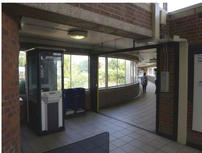
View looking North West from Booking Hall towards existing Overbridge.
